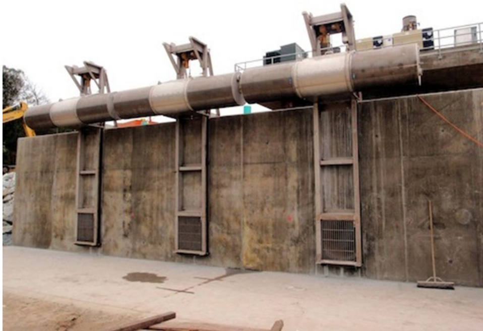
Figure 3-14: Retrievable Cylindrical Wedgewire Screen at Salinas River Diversion Dam near Monterey, CA (Courtesy ISI)
