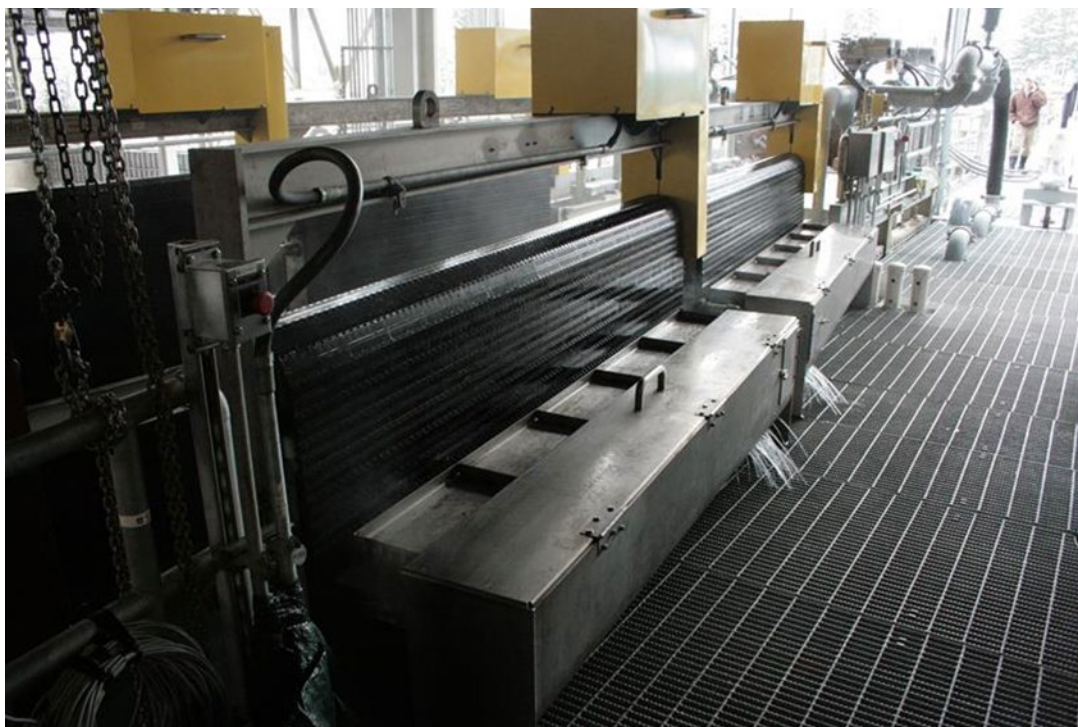
Figure 3-9: Hydrolox Screens with a Water Backwash at the Cowlitz Falls North Shore Collector on the Cowlitz River, Washington (Courtesy Tacoma Power)
