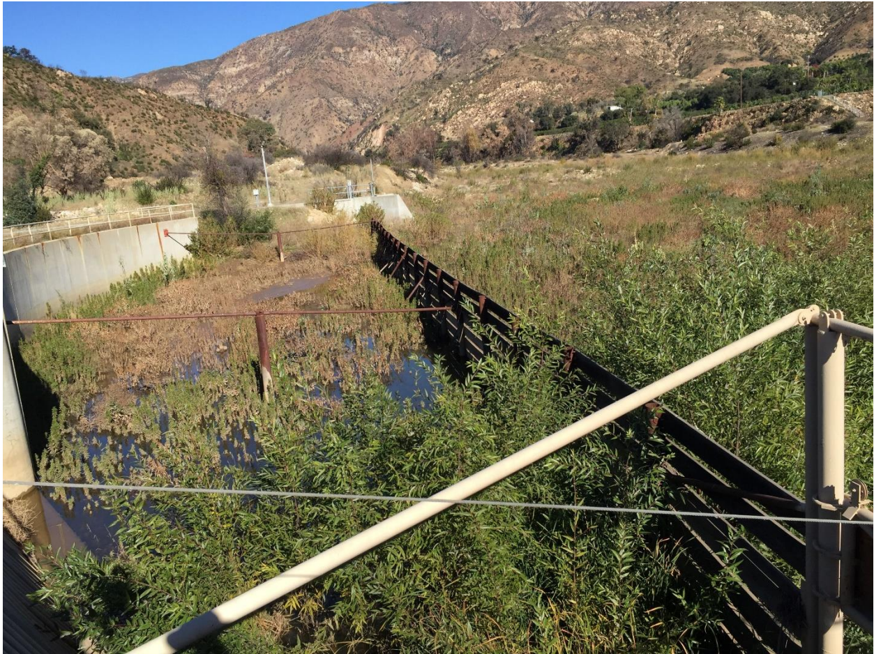
Photograph 3. View looking northwest, while standing on the bridge over the spillway, of the forebay area and timber debris fence upstream of the Diversion Canal Headworks.
