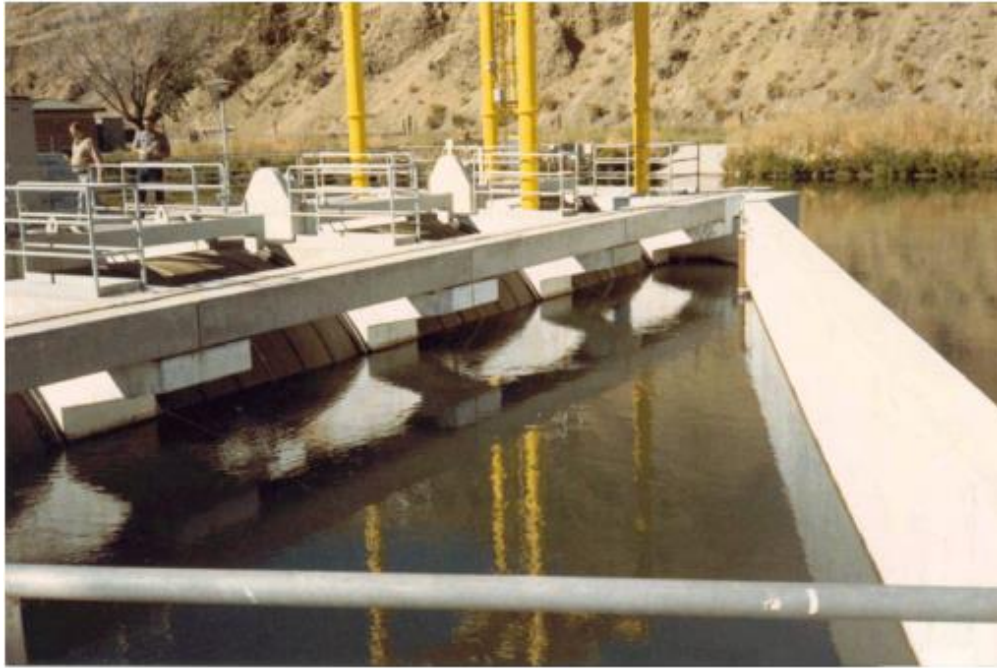
Figure 14. Drum Screens at Roza Diversion (from USBR “Fish Protection at Water Diversions”, 2006)
