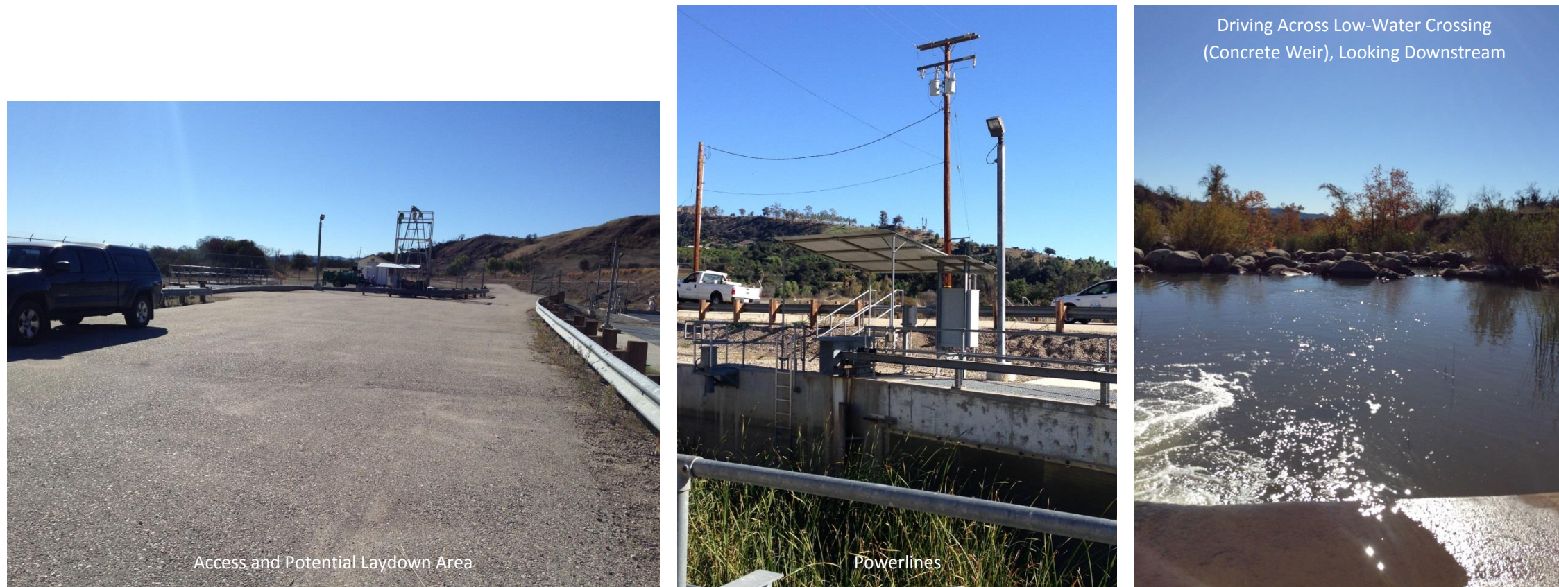
Figure 11. Site Visit Photo Summary, Sheet 2 of 2
