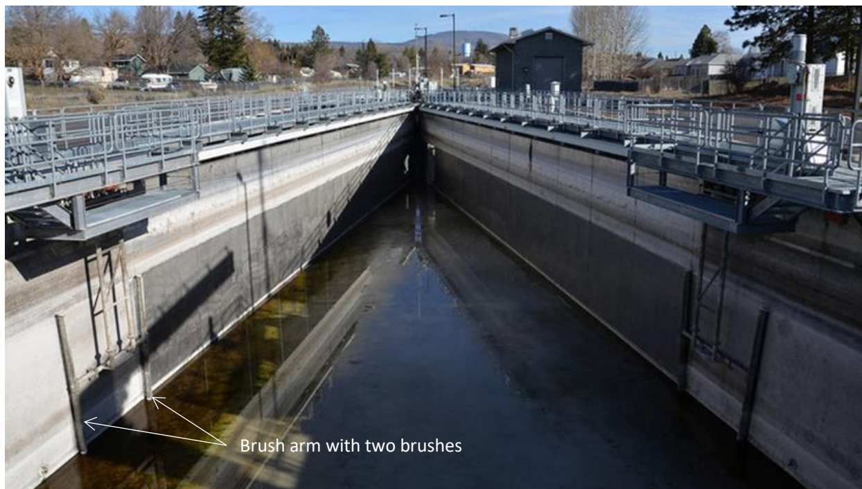
Figure 3-4: V-screen brush with Two Brush Arms per cleaning system at the A-canal Diversion Klamath River, OR (Courtesy Bureau of Reclamation) ( https://www.flickr.com/photos/usbr/16411346396 )
