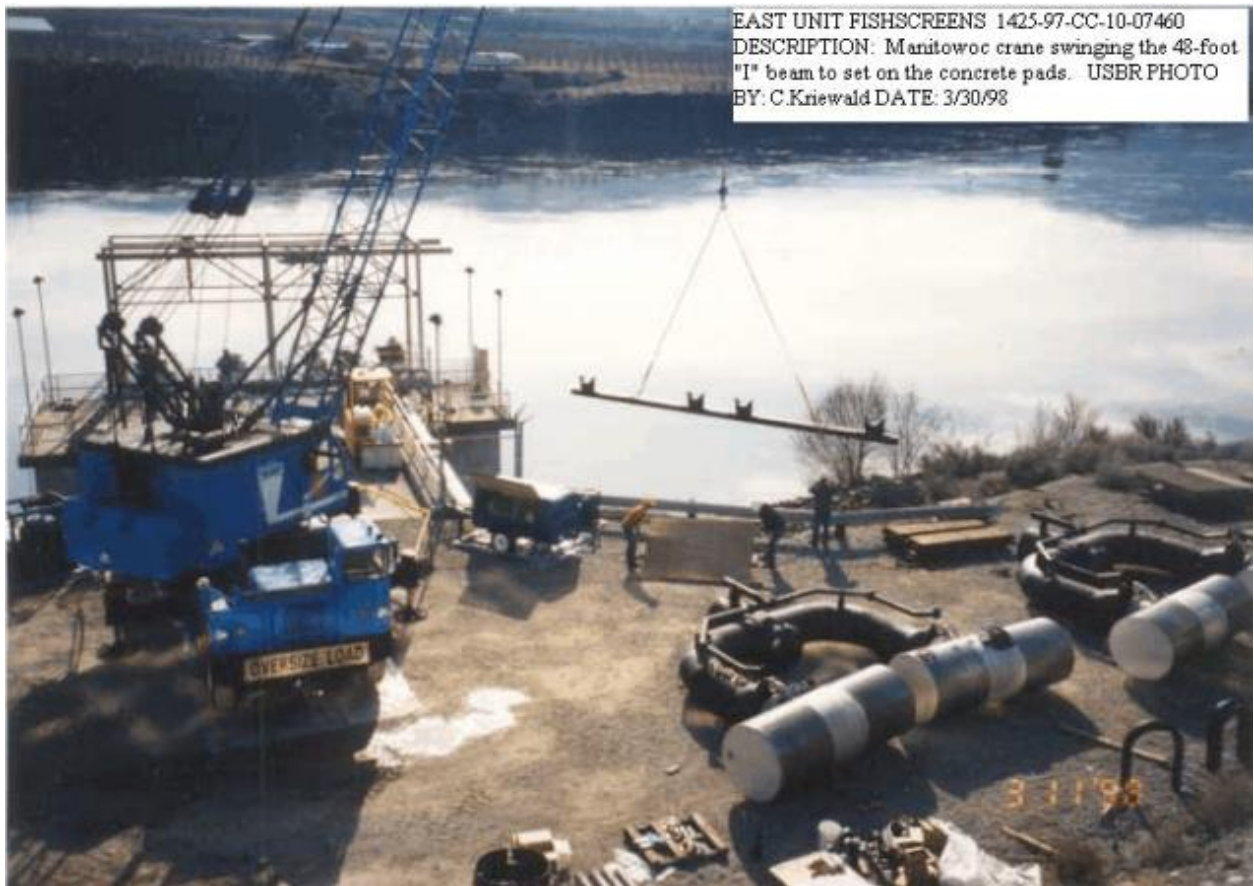
Figure 16. Installation of Cylindrical Tee Screens, East Unit Pumping Plant, WA (from USBR "Fish Protection at Water Diversions", 2006)
