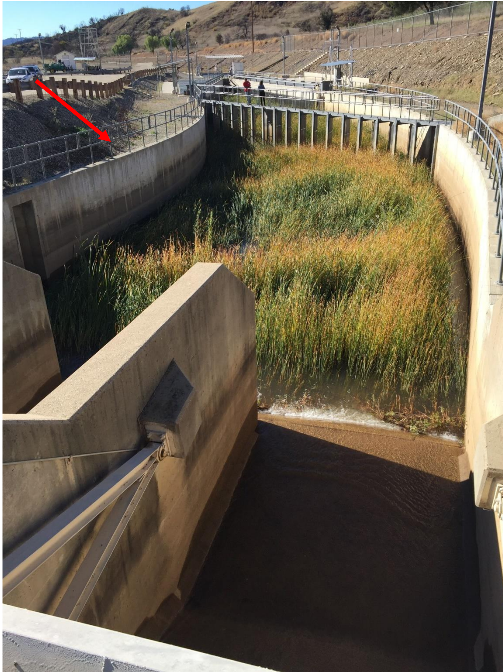
Photograph 4. View looking southwest down into the Diversion Flume area. The east side of the Diversion Flume would be excavated to implement Alternative 4.
