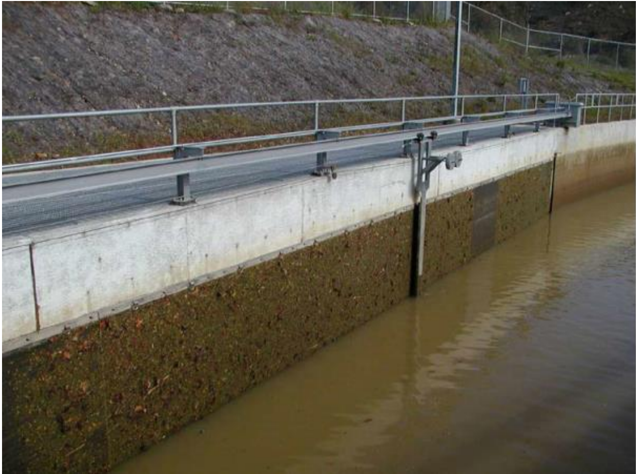
Photograph 1. View looking north of Robles Fish Passage Facility V-screens (west side of the Fish Screen Channel) of debris material that has accumulated on the screens.
