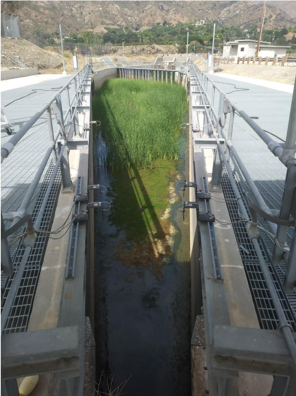
Photograph 2. View looking northwest standing at the downstream end of the Fish Screen Structure at the Fish Screen Channel.
