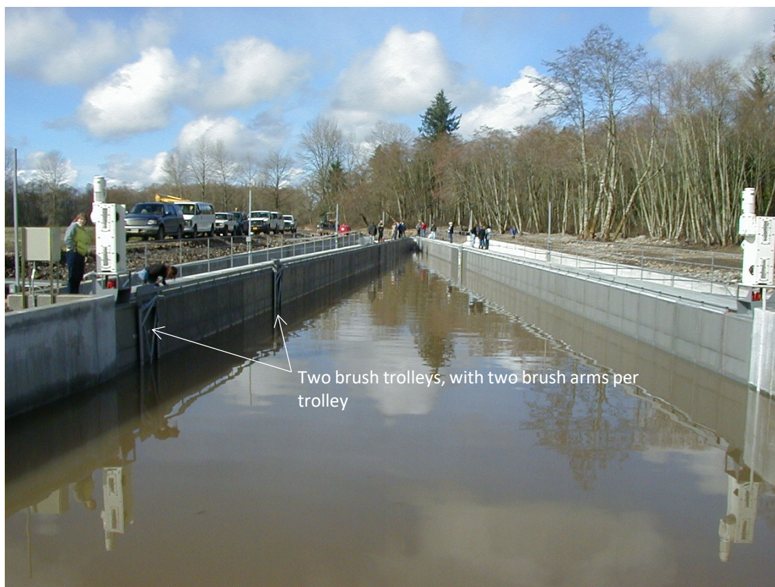
Figure 3-2: V-screen with Two Brush Systems per Side on the Santiam River, OR (Courtesy Santiam Water Control District)
