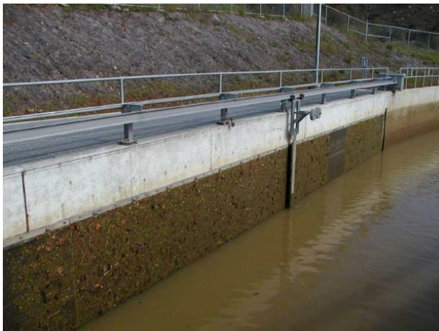
Figure 13. Typical Debris, Pre-Fire
