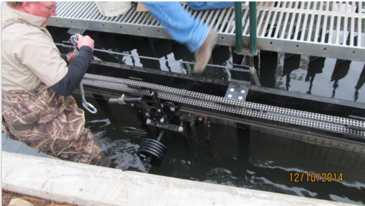
Figure 3-1: Chain Drive at the North Fork of the Sprague River, OR
