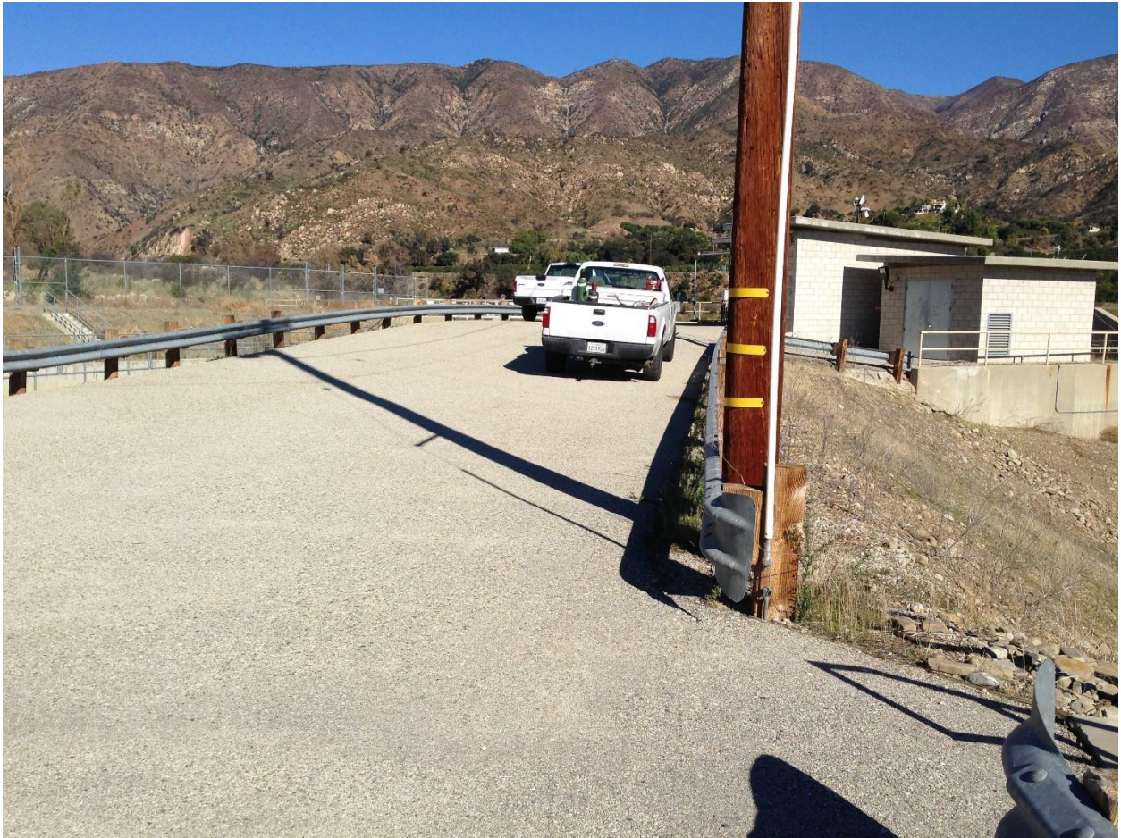
Photograph 5. View looking north, of the paved road above the east side of the Diversion Flume and Fish Screen Channel area. Excavation would occur in this area to implement Alternative 4.
