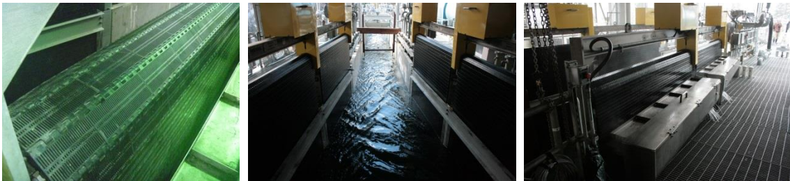
Figure 13. Traveling Screen System: a) Close Up, b) Upstream, c) Downstream (Cowlitz Falls Dam Fish Collection Facility)
